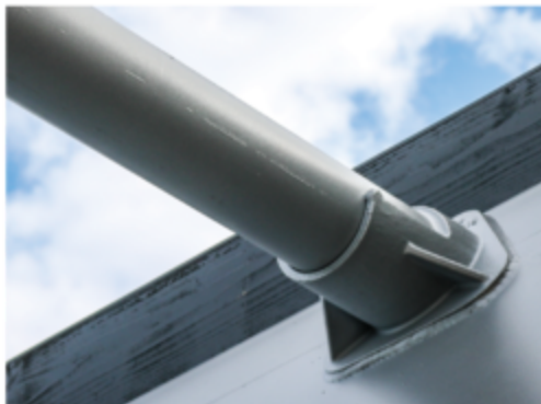
Cast Steel Mountings Round hopper cross members attached to sidewall with cast steel mountings.
